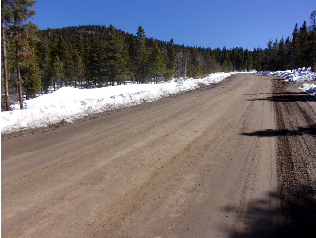
Virginia Canyon Road Conditions looking South with the subject property on the left.
