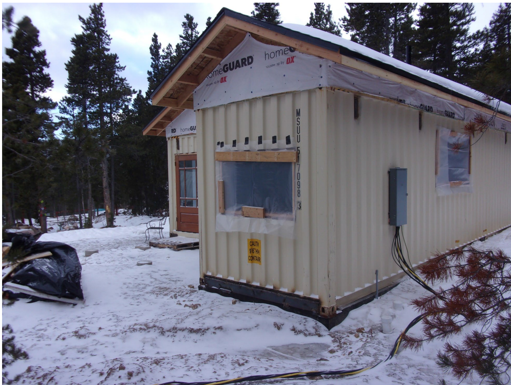
105 Conestoga Exterior Photos
