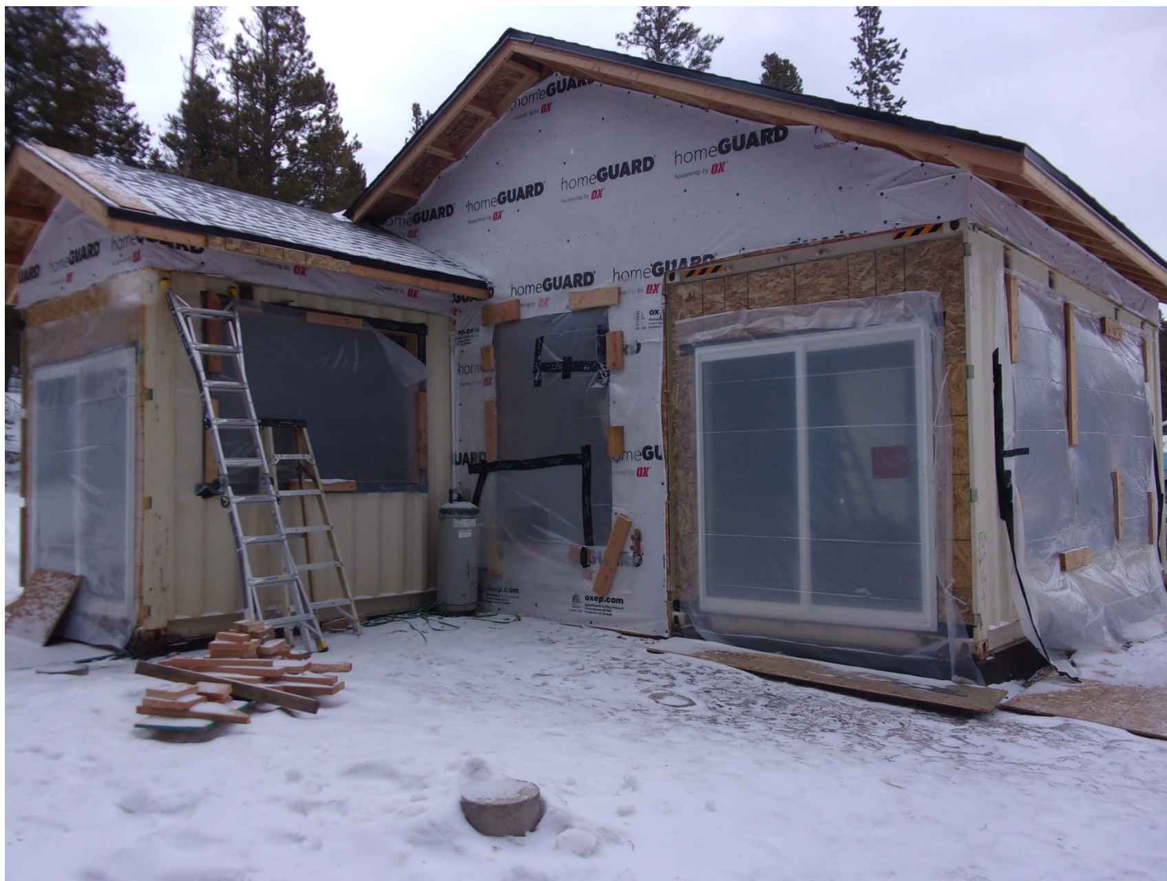
105 Conestoga Exterior Photos
