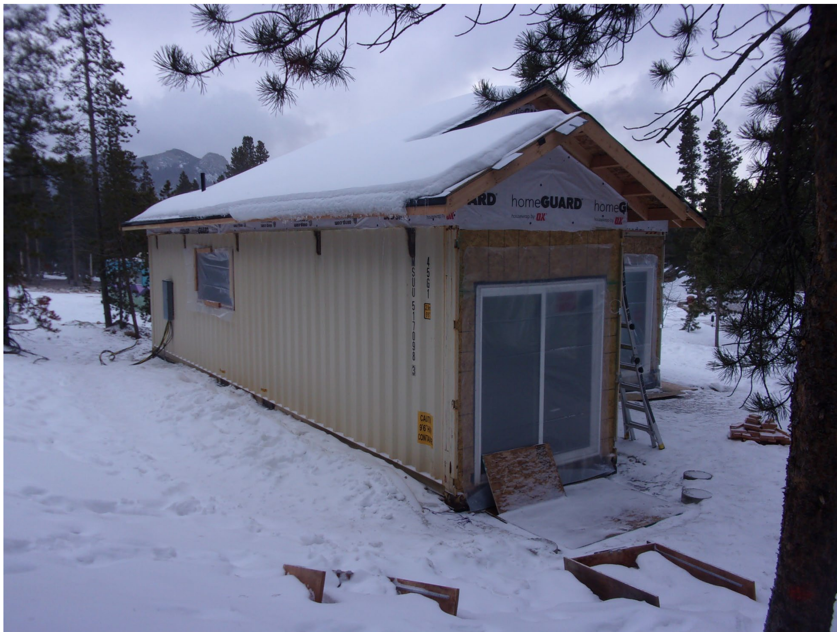
105 Conestoga Exterior Photos
