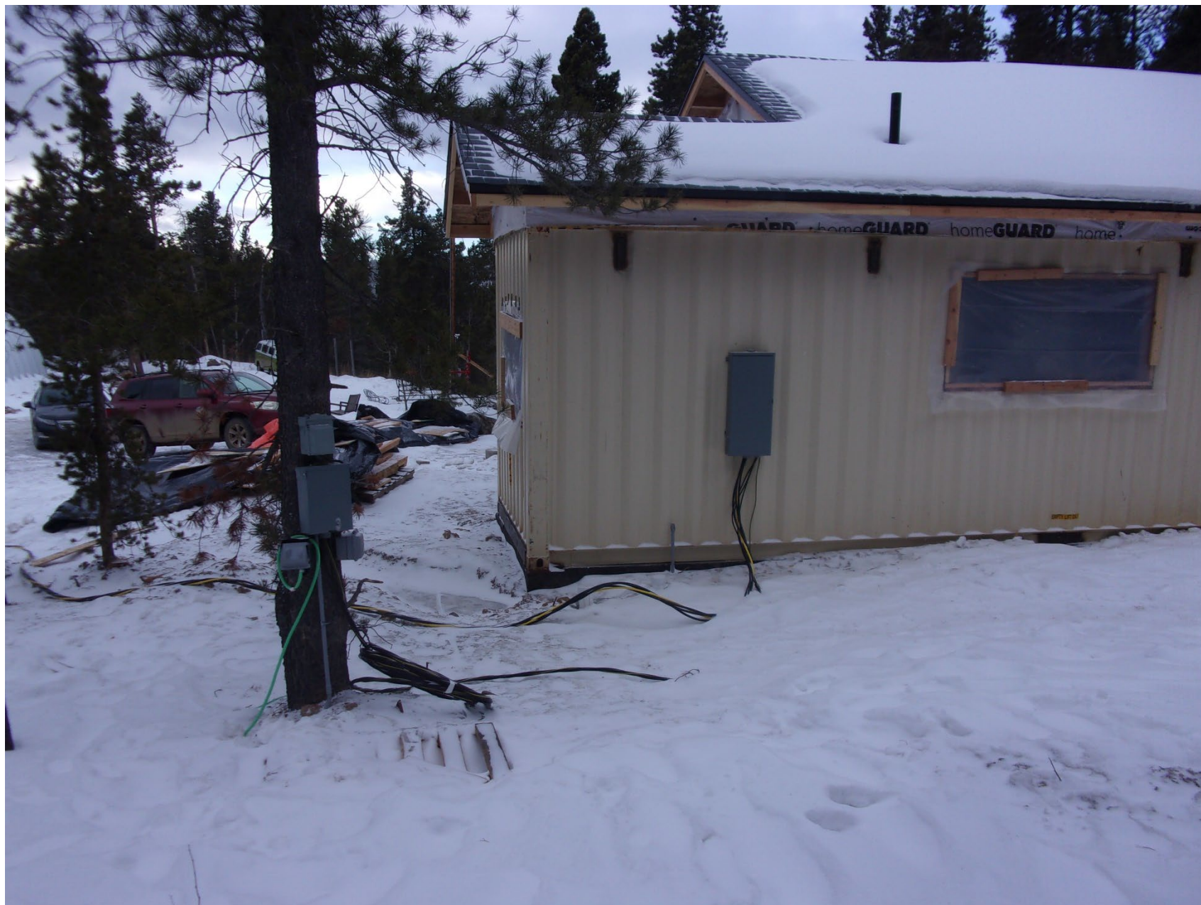
105 Conestoga Exterior Photos
