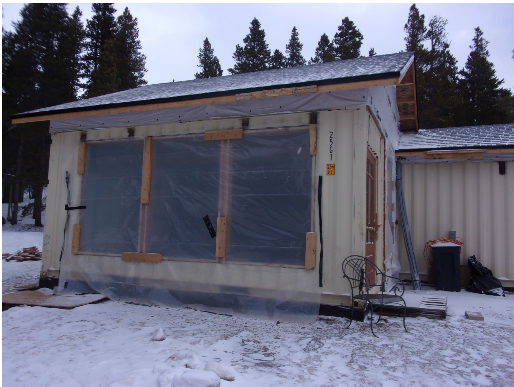
105 Conestoga Exterior Photos
